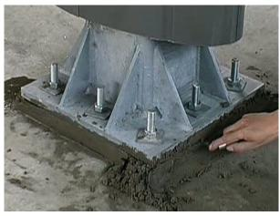
After installation put a shrink free concrete under the base plate!
