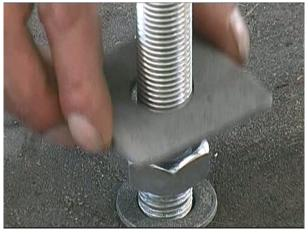
Put the square plates (60x60x5 mm) on top of the bolts
